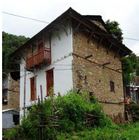
Vernacular stone house with appropriate construction details that survived the earthquake
